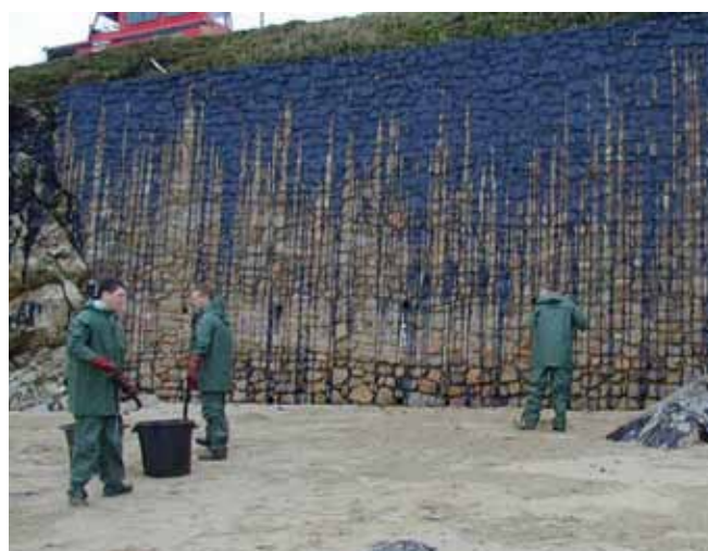
▲ Figure 15: Heavy oiling of a sea wall following a storm tide.
